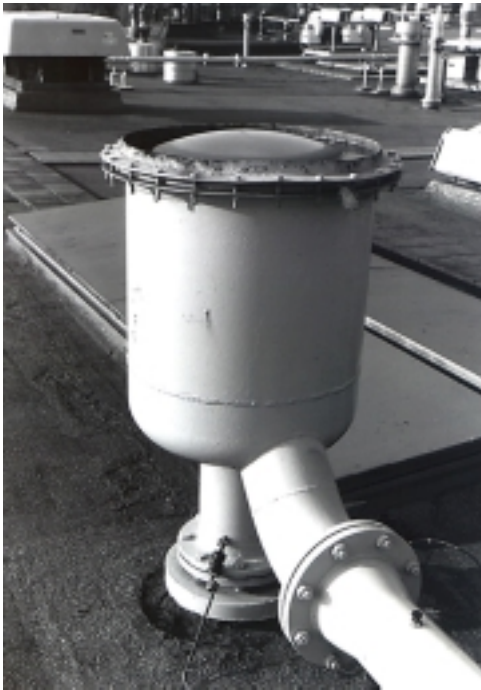
Fig. 7. Explosion diverter
